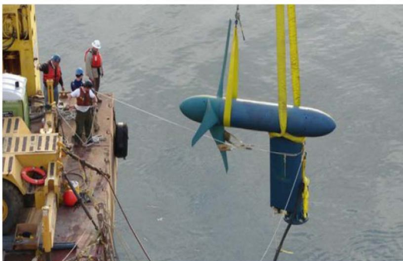
Figure 1: Verdant Power's Free Flow Kinetic Hydropower System, an axial-flow tidal turbine, is lowered into the East River, New York. Photo credit: Verdant Power, Inc.
