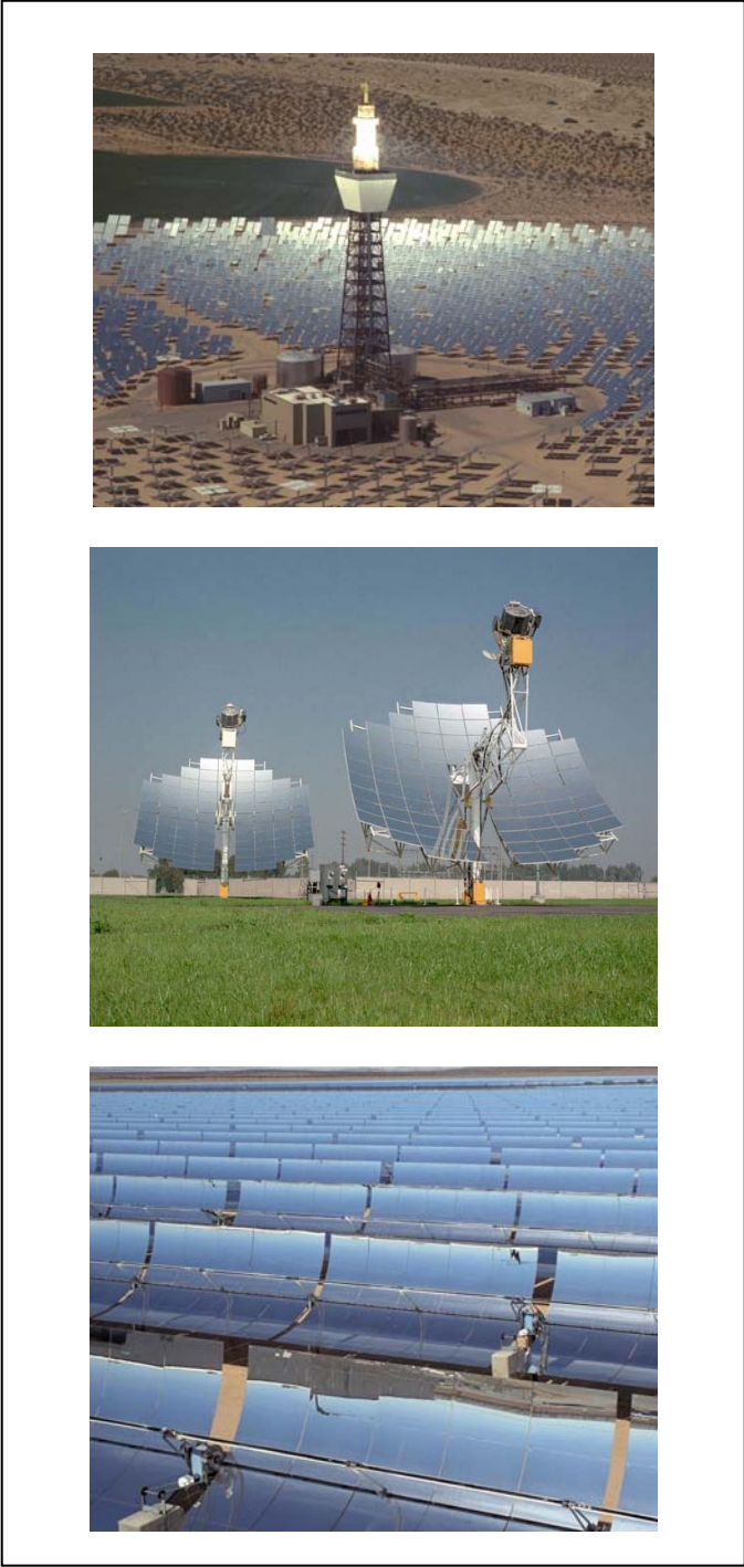
Figure 1. Solar tower, dish, and trough power plants
