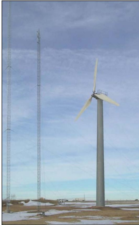
**Figure 1. Modified Micon 65 Turbine (Shown with SERI-8 Blades)**
